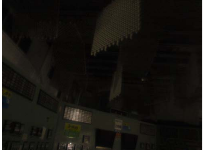
Picture2: Situation of Central Control Room of Units 1 and 2
