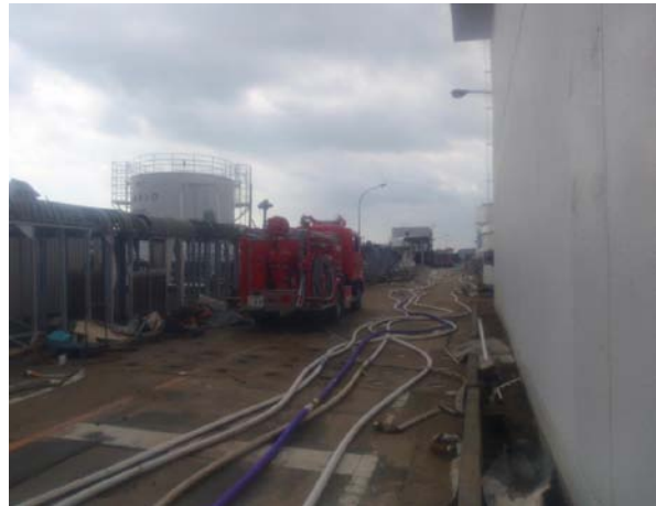
Picture 6 : Situation from Protection Control Gate of Units 1 and 2 towards Unit 3
