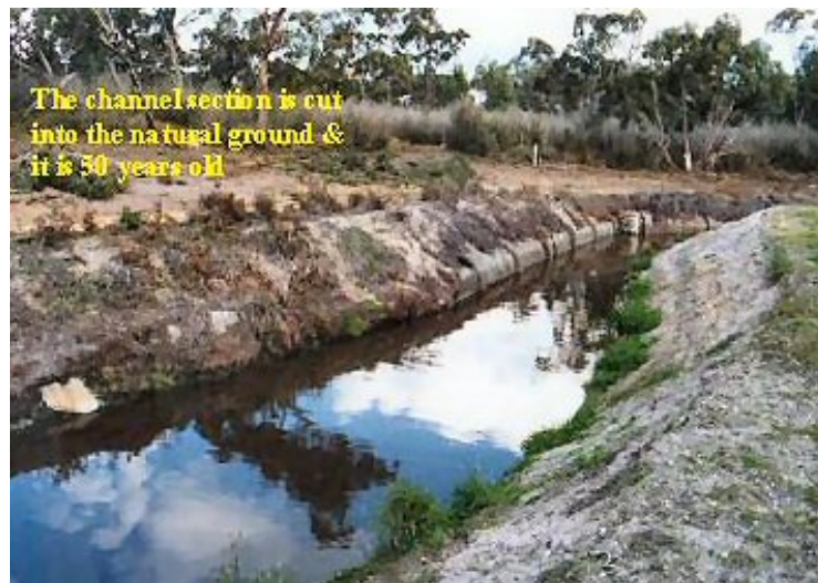
Figure 32: The open channel regional outlet sewer in Gippsland [Gippsland Water, 2004b]
