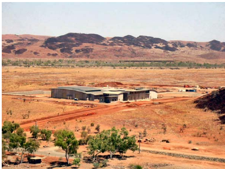
Figure 29: Harding Dam UF water treatment plant [Photograph courtesy of Z. Tonkovich; Zenon Australia]
