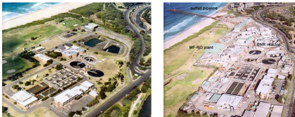
Figure CE3.1: Wollongong existing STP (left) and current constructions (right)
