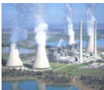
Figure 61: Bayswater and Liddell Power Stations.
