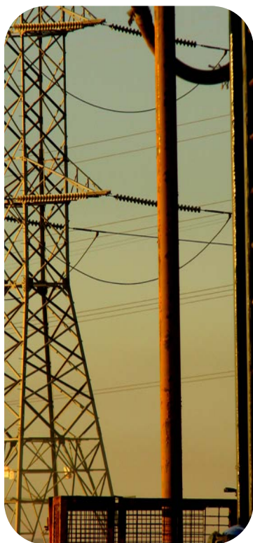
Watson Drilling casing operations at Port Augusta, with 275kV transmission line in background.
