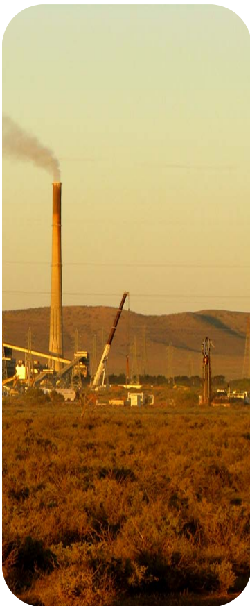
Port Augusta power station (above) with Theoden 2 drill site in right foreground.
