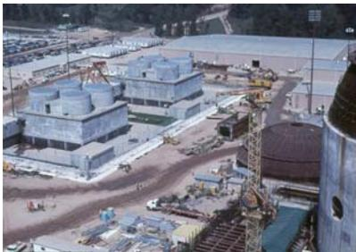
▶ *The Vermont Yankee nuclear plant uses two mechanical type cooling towers during normal operation and two special cells in one of those towers in event of an accident.*
