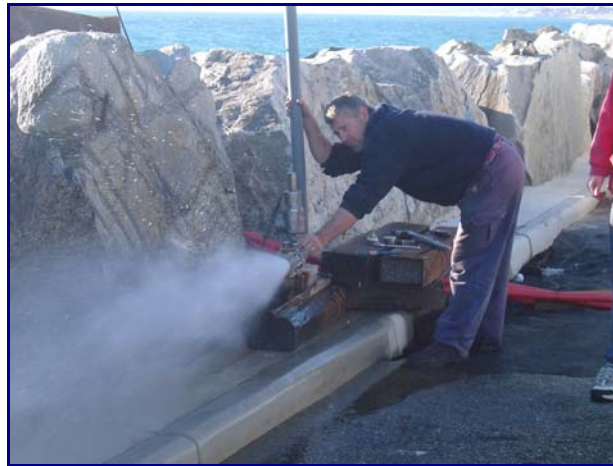
Figure 2.9 Delivery of pressurised seawater ashore
