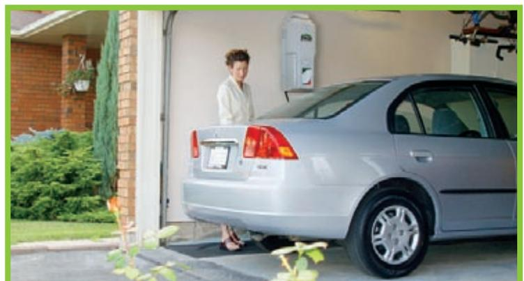
Figure 2. Phill Provides CNG Refueling inside Residential Garages
