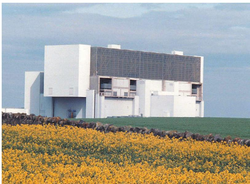
Torness is located on the East Lothian coast 35 miles from Edinburgh. The nuclear power plant comprises two Advanced Gas Cooled Reactors (AGR). The two reactors are practically identical. The combined net power output is 1250MW electricity, which represents around 12% of the current generation capacity in Scotland.
