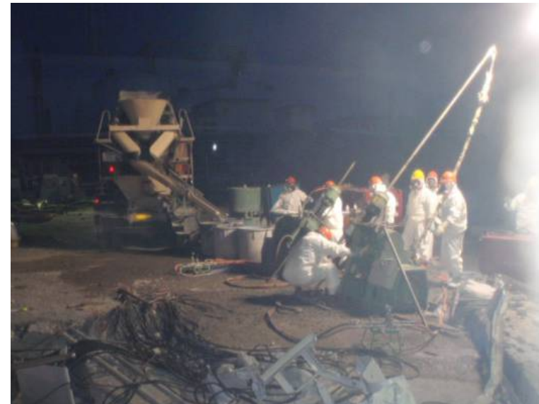
Coagulant injection to stop outflow
