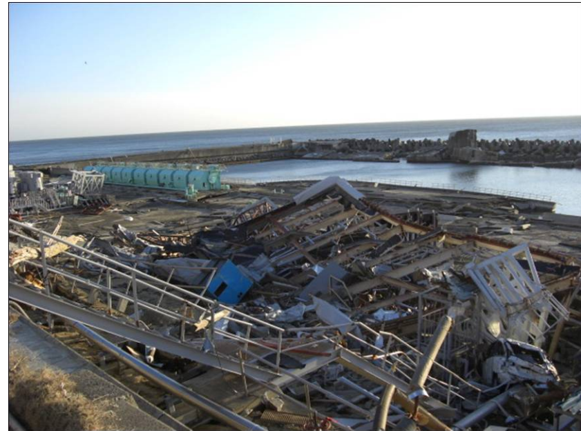
Unit 5,6 Intake Screen Area
