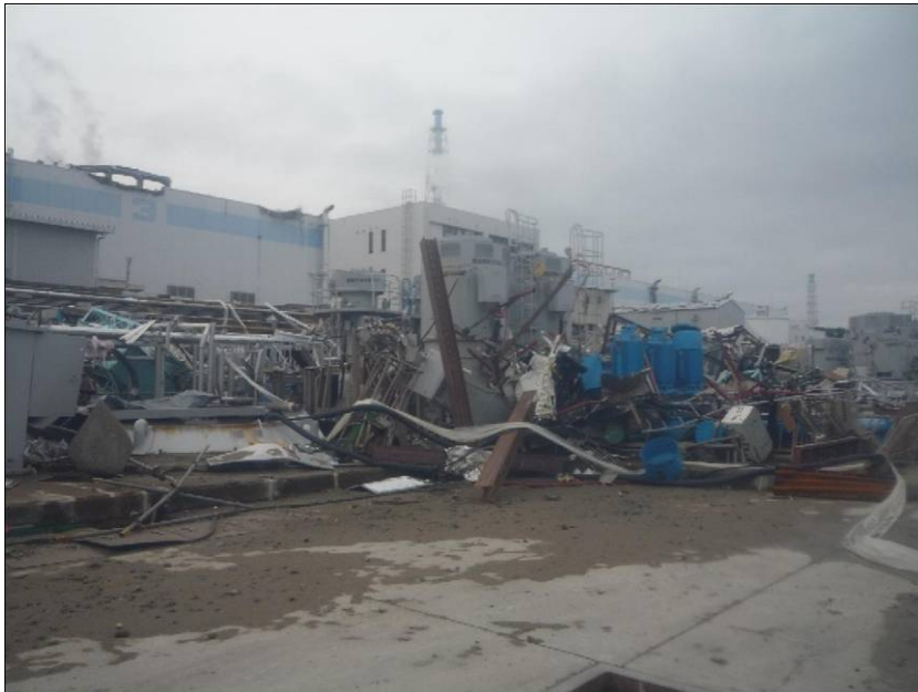
Unit 3 Sea Pump Area
