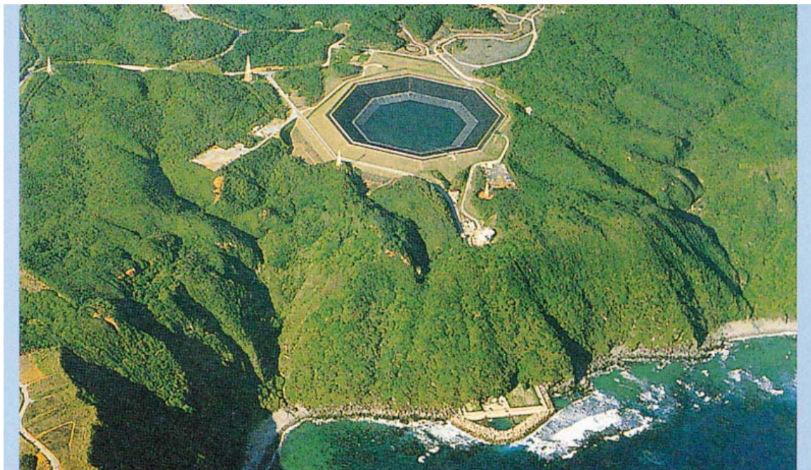
Figure 6 Pilot Seawater Pumped-storage Power Plant, Okinawa Pref. in Japan. The octagonal shape shows the upper dam. The outlet of the tailrace is surrounded by tetra-pods for protection from waves. The picture is from the 1998 Hitachi Review.
