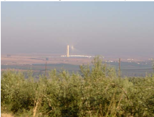
A view of PS10 concentrating solar radiation in the stand-by position ready to aim the solar receiver
