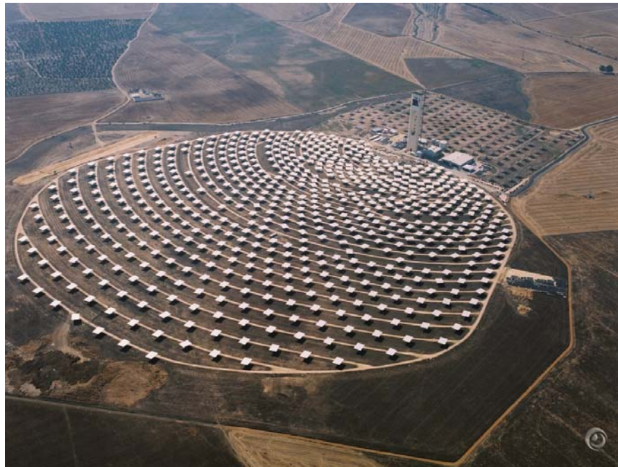
Aerial view of PS10 11MW solar plant
