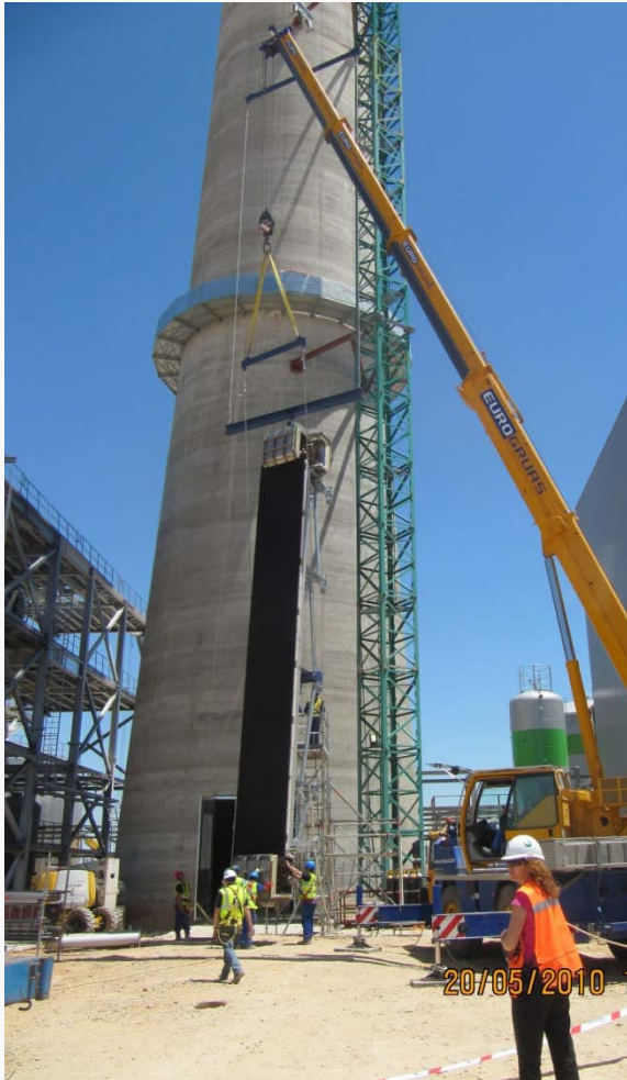
Receiver panels lifting operation
