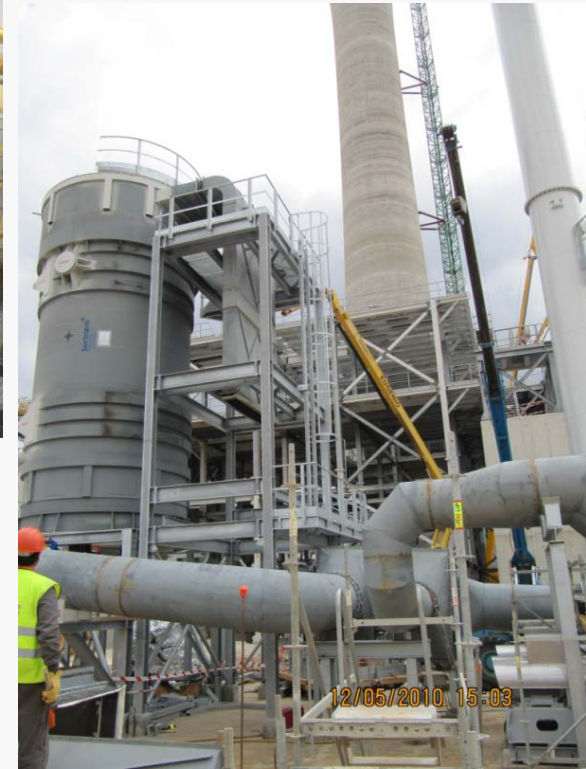
Gas fired salt heater erection
