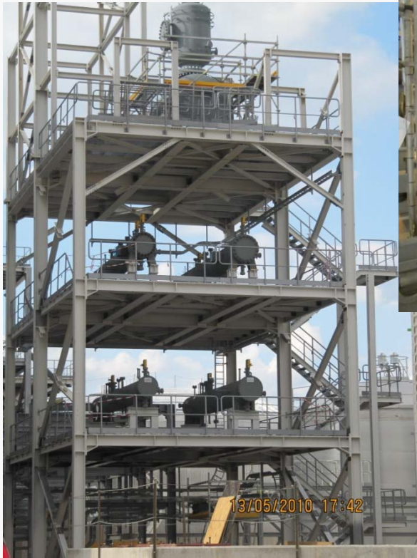
Structure building for deaerator and feedwater preheaters
