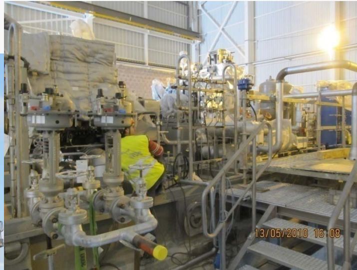
Detail of progress of steam turbine mechanical erection
