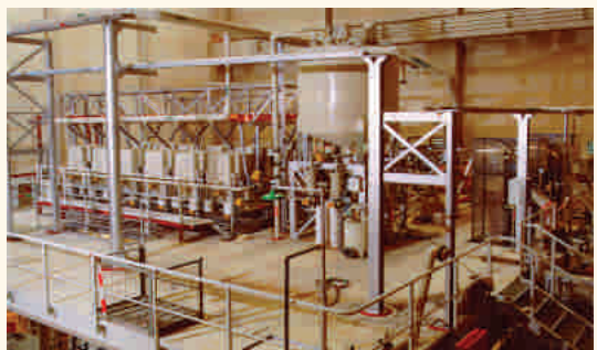
Electrowinning section of Electric Fuel's regeneration plant in Bremen, Germany
