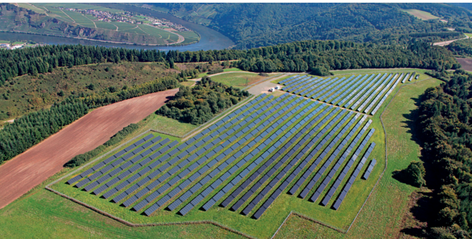
Photovoltaics on a grand scale: the solar power plant "Mehringener Höhe".
