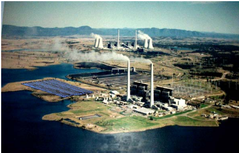
Figure 5. Liddell Power Station with an impression of the 25MWe CLFR array located at the proposed site adjacent to the plant.
