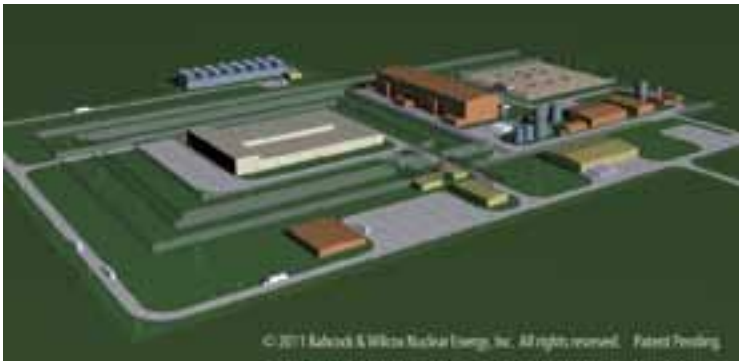
Conceptual SMR site plan with two below-ground reactor modules in the nuclear island (left side, white building).
