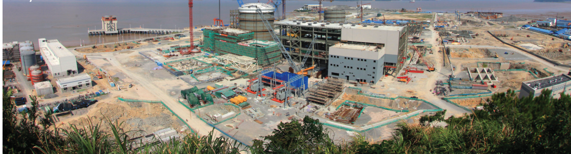
An AP1000 under construction at Sanmen, China , October 2011
