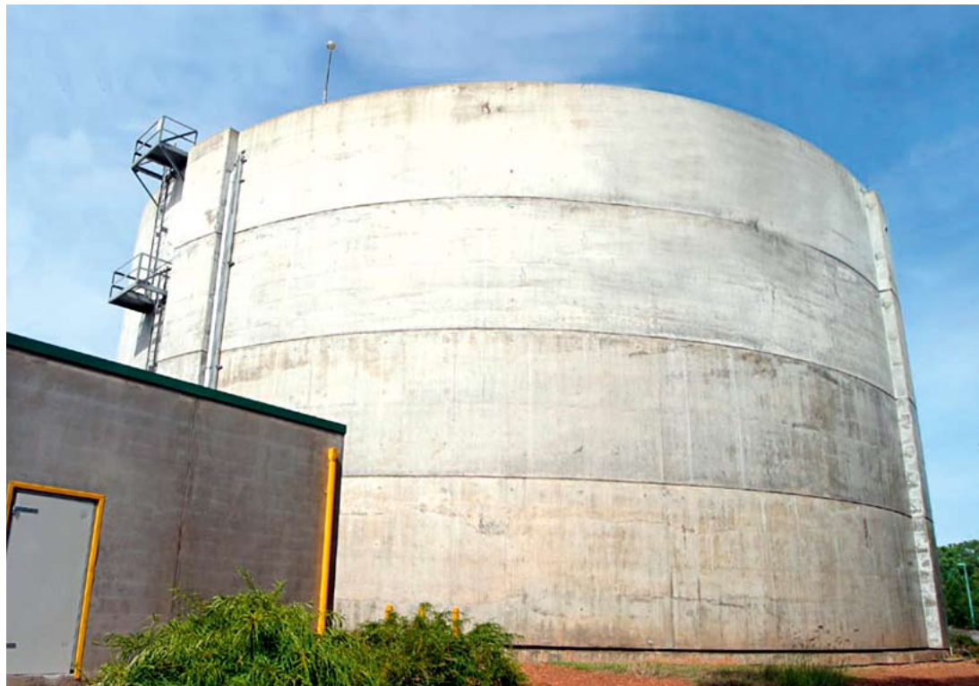
Charles Darwin University, chilled water storage tank
