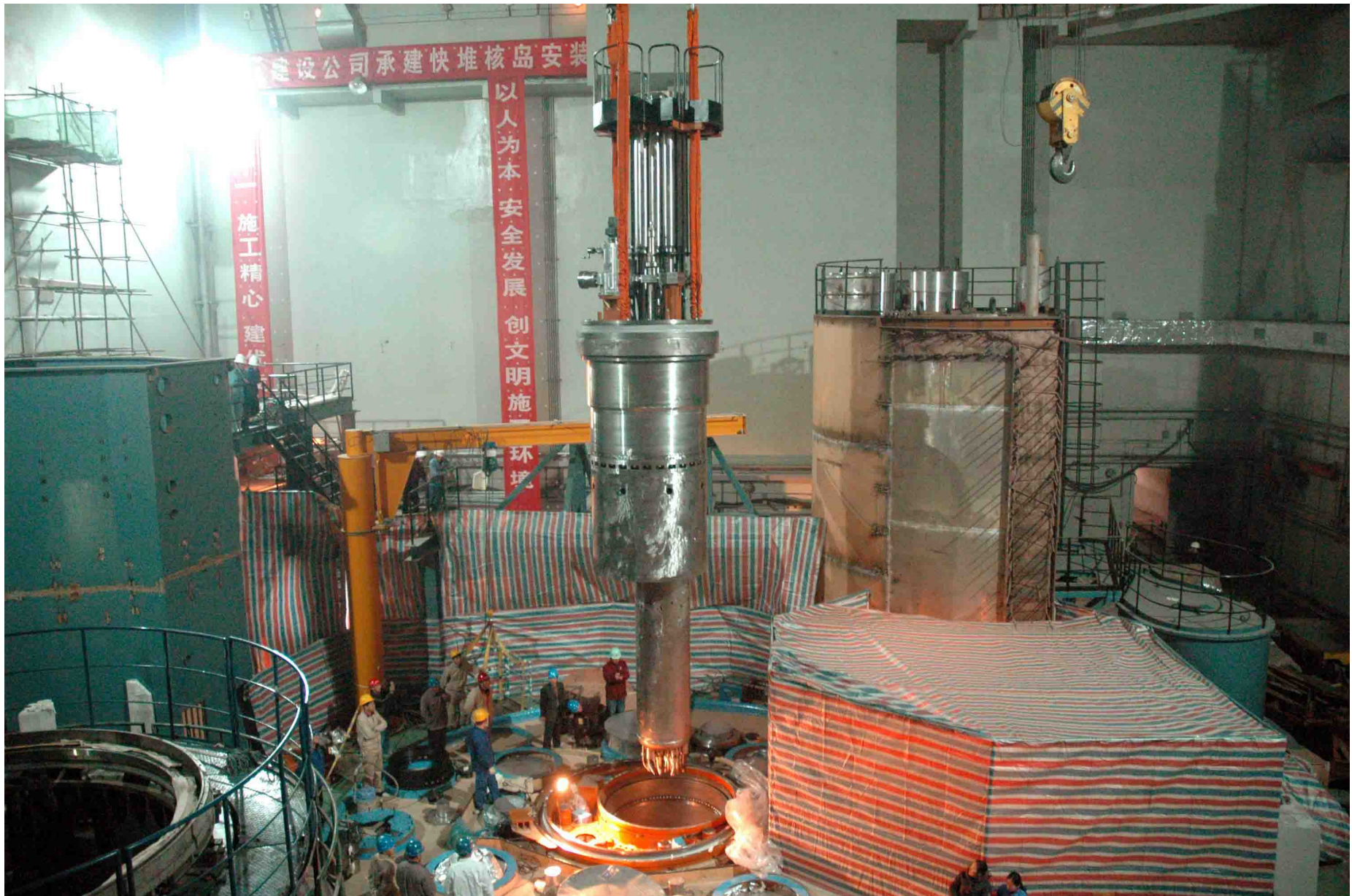
Small rataling plug under installation (2003.03.22)
