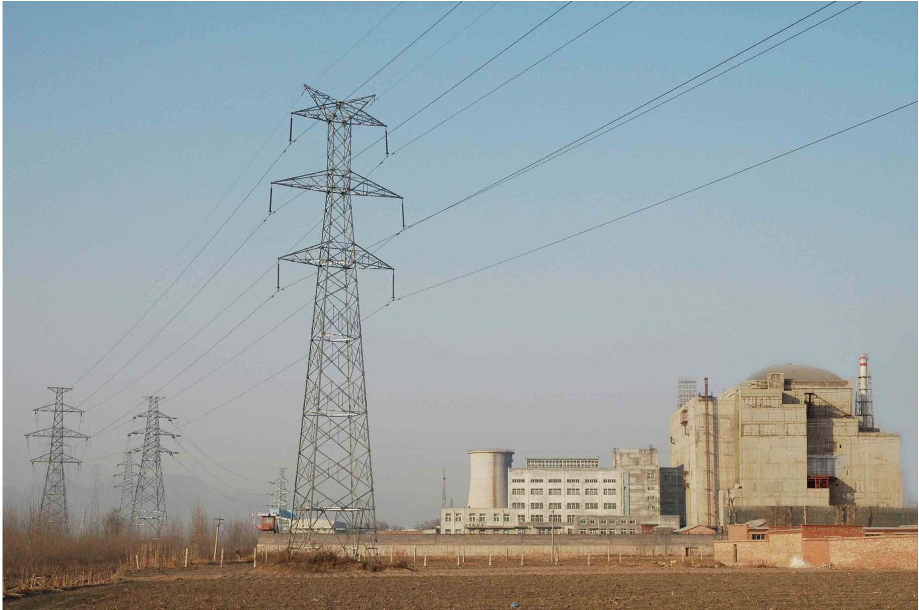
National Grid comes to the site (2007.01.28)
