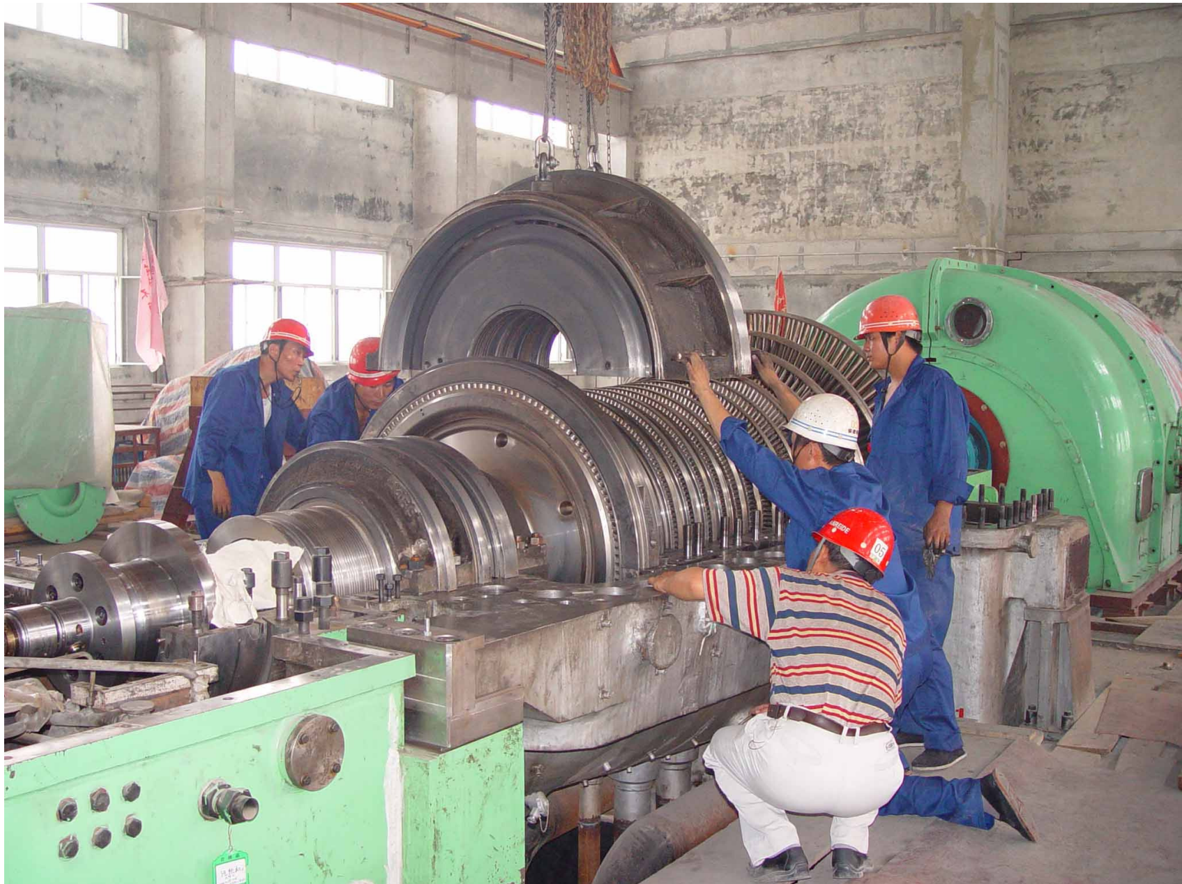
Turbine under installation (2005.07.21)
