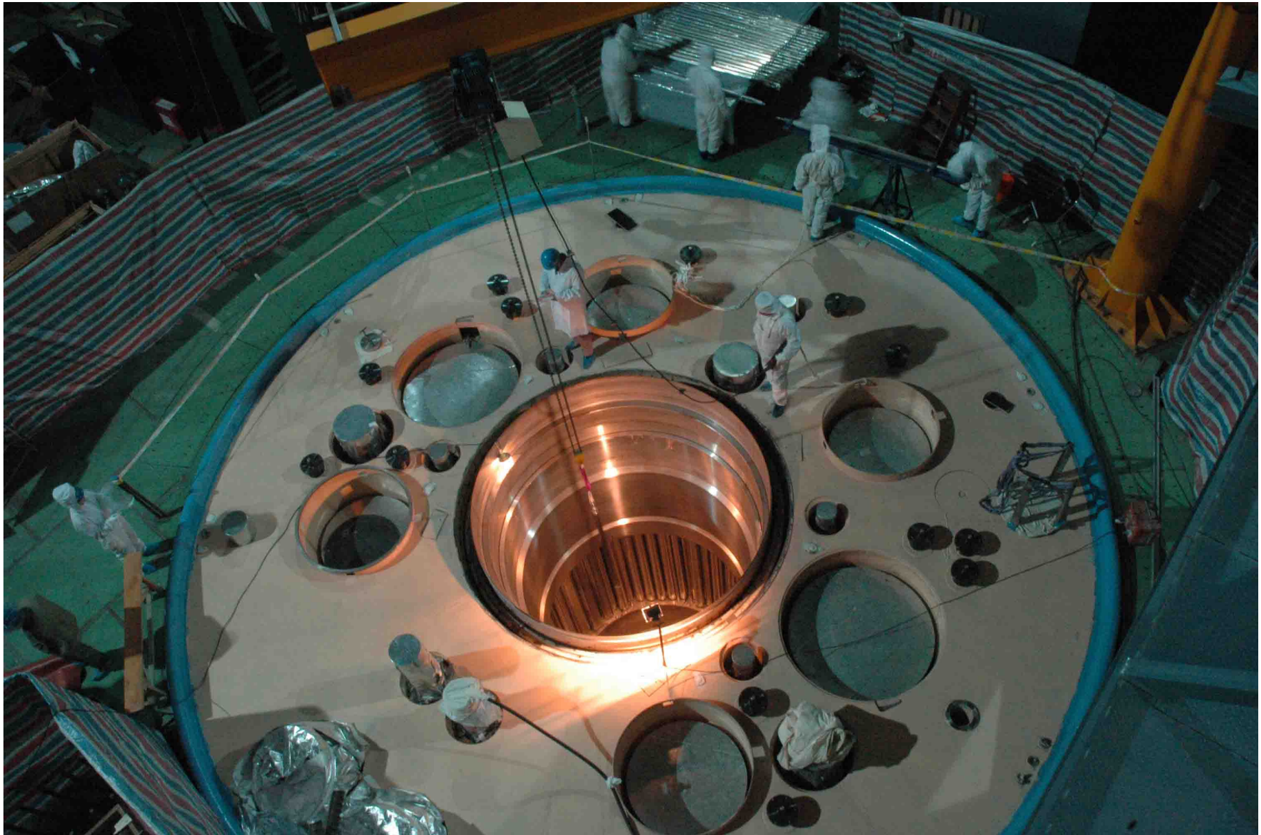
Core Reflector Subassembly moving to the core (2008.02.26)
