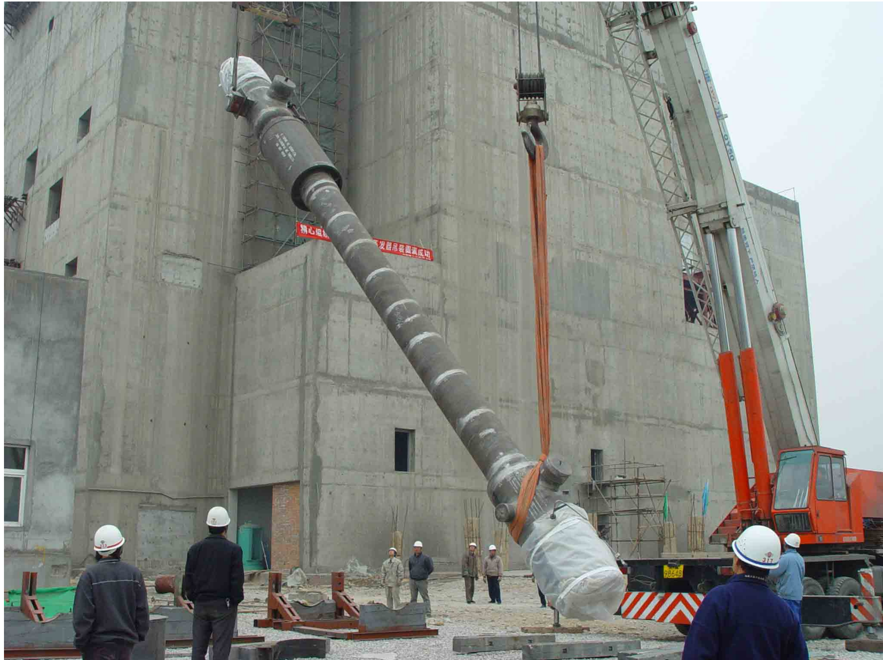
Evaporator Moving to Reactor Building (2005.03)
