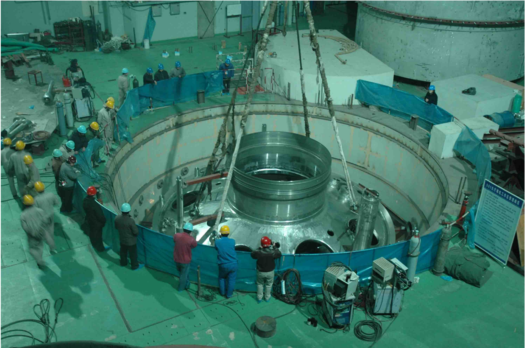
Reactor block and Main Vessel under Installation
