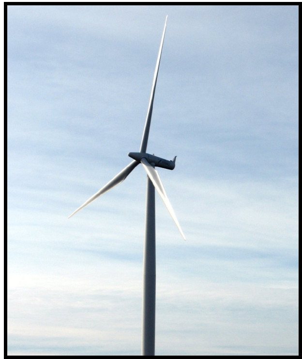
POLLUTION-FREE: WIND TURBINE ON WOLFE ISLAND. Photo by Mike Buckthought.
