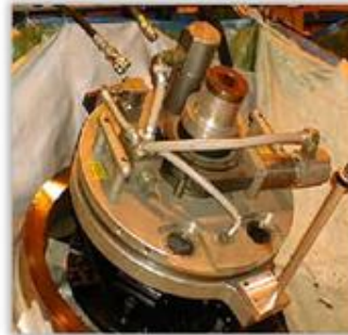
On-site narrow space groove processing
