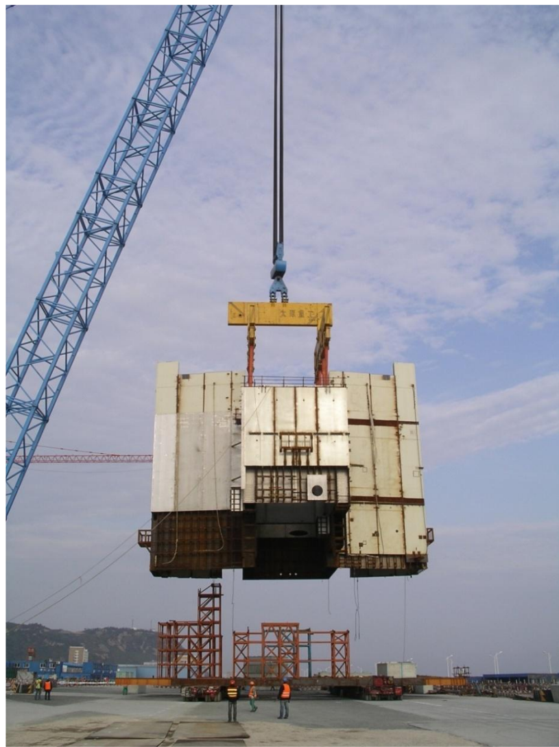
March 27, 2010: CA01 lift, rotation and lowering into CV
