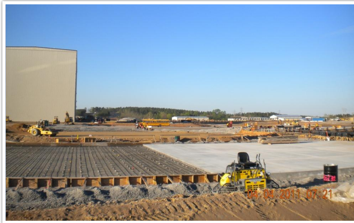
Pad 43, Pad 32A&B Rebar Staging & Fabrication
