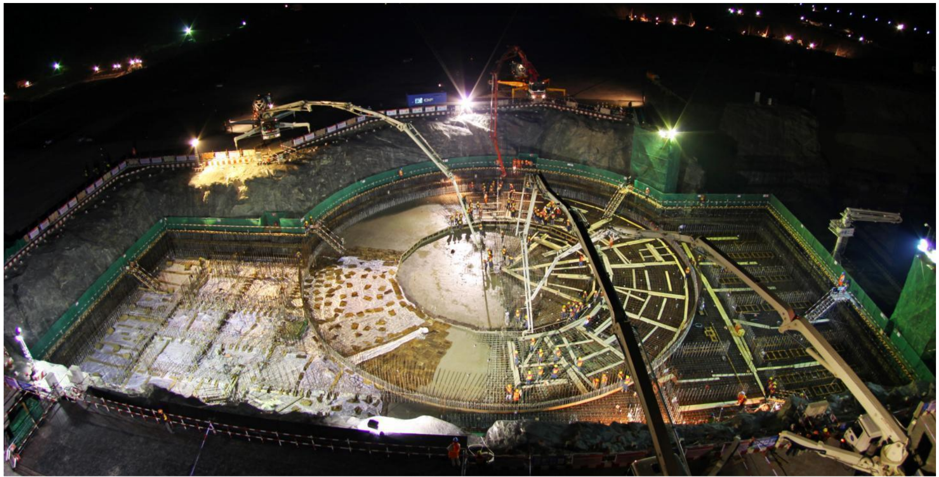
March 2009: First Nuclear Concrete
