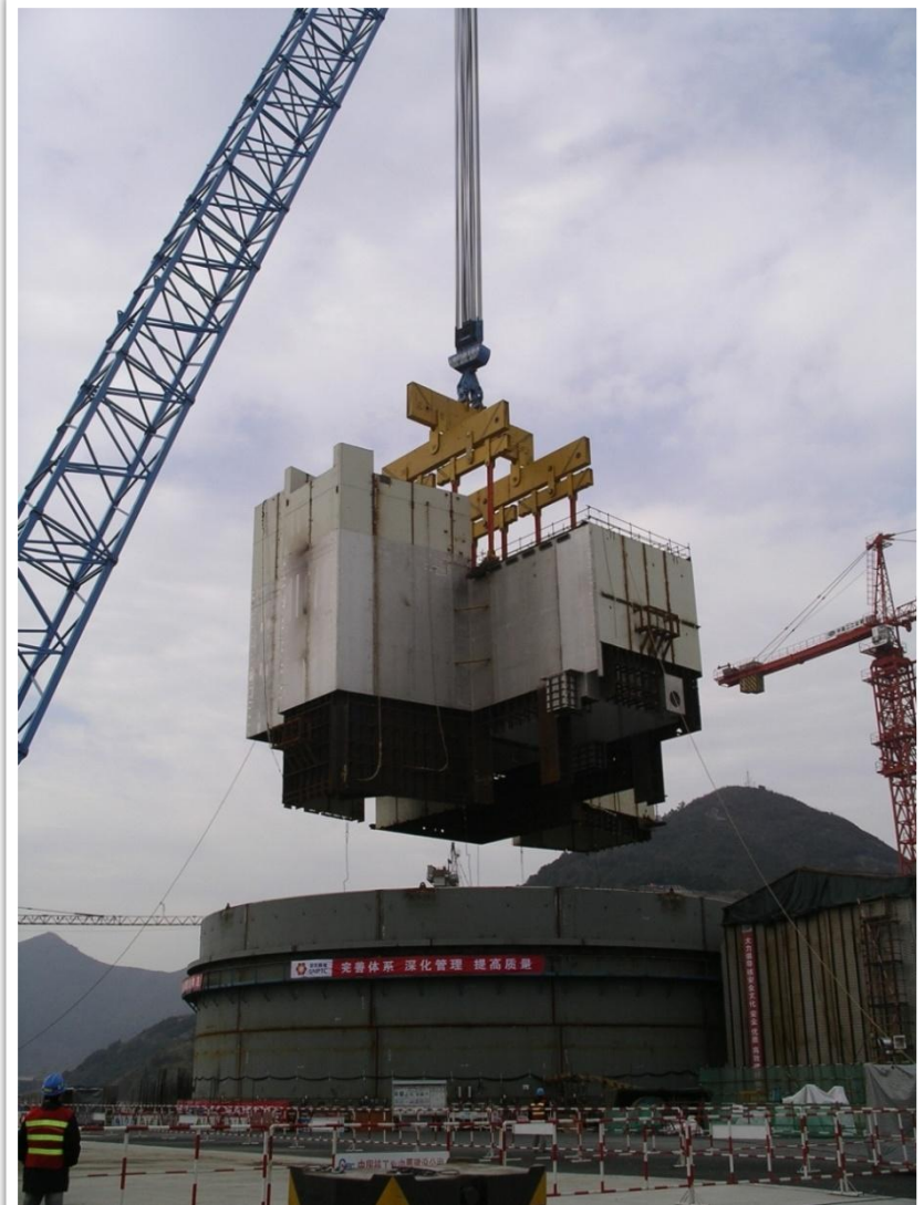
March 27, 2010: CA01 lift, rotation and lowering into CV
