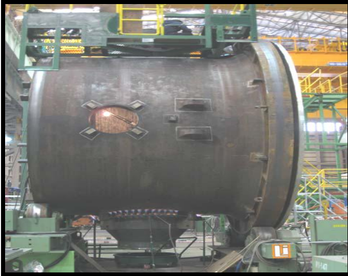
RV Outlet Nozzle welding of Upper Shell – Unit 2
