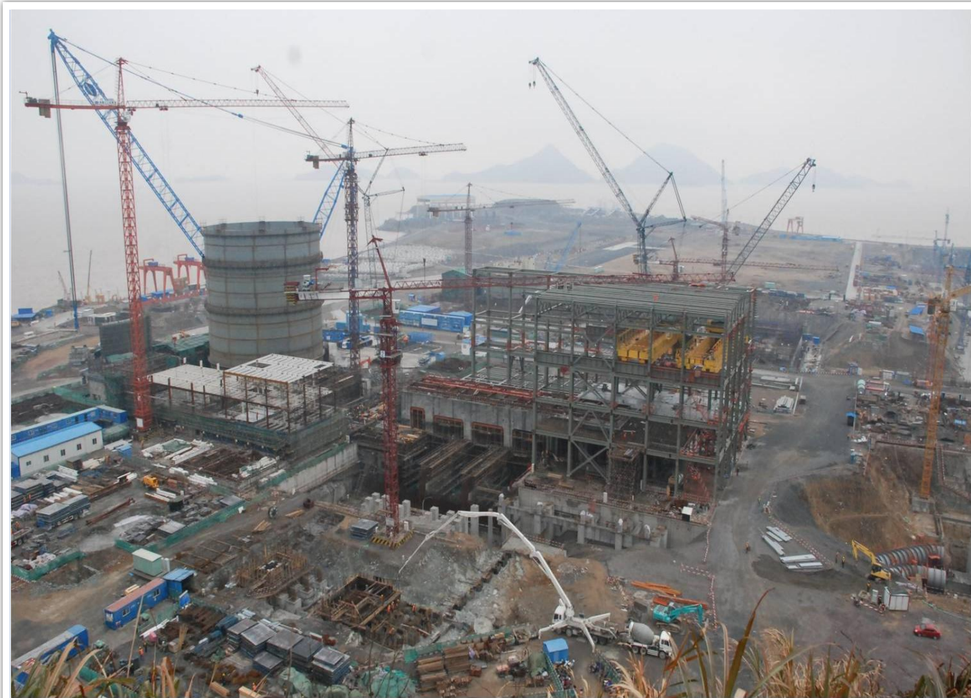
January 2011: Sanmen Site Overview
