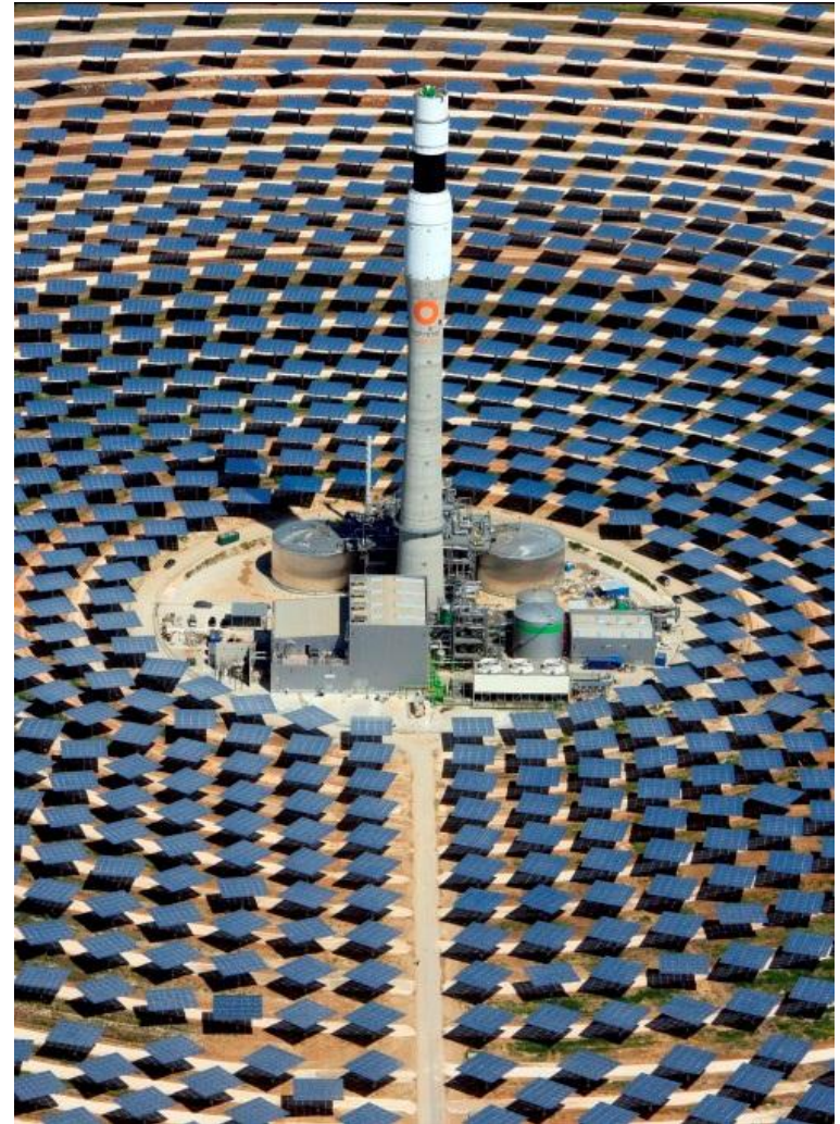
Aerial View of Gemasolar (April 2011)
