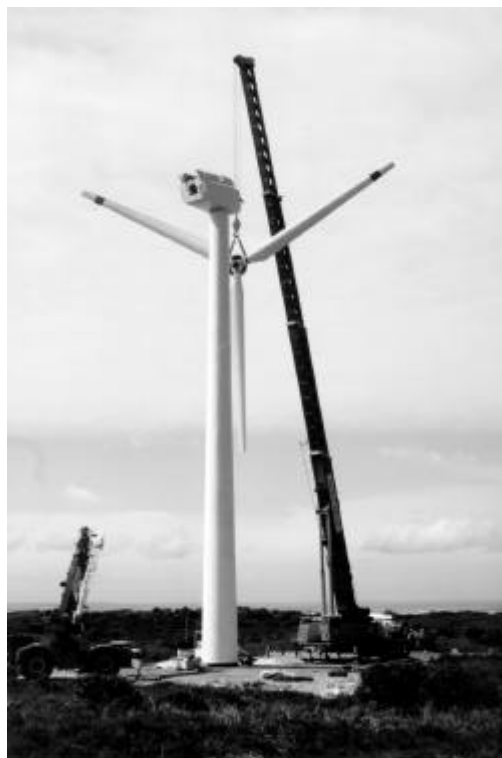
Figure 4. One of the turbines at Ten Mile Lagoon being assembled; photo shows rotor being lifted into place.
