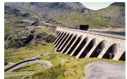
Figure 26.6. Llyn Stwlan, the upper reservoir of the Ffestiniog pumped storage scheme in north Wales. Energy stored: 1.3 GWh. Photo by Adrian Pingstone.
