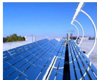
Figure 6.19. A combined-heat-and-power photovoltaic unit from Heliodynamics. A reflector area of 32 \text{ m}^2 (a bit larger than the side of a double-decker bus) delivers up to 10 kW of heat and 1.5 kW of electrical power. In a sun-belt country, one of these one-ton devices could deliver about 60 kWh/d of heat and 9 kWh/d of electricity. These powers correspond to average fluxes of 80 \text{ W/m}^2 of heat and 12 \text{ W/m}^2 of electricity (that's per square metre of device surface); these fluxes are similar to the fluxes delivered by standard solar heating panels and solar photovoltaic panels, but Heliodynamics's concentrating design delivers power at a lower cost, because most of the material is simple flat glass. For comparison, the total power consumption of the average European person is 125 kWh/d.
