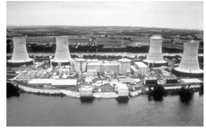
Figure 24.4. Three Mile Island nuclear power plant.
