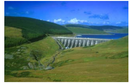
Figure 8.1. Nant-y-Moch dam, part of a 55 MW hydroelectric scheme in Wales. Photo by Dave Newbould, www.origins-photography.co.uk .
