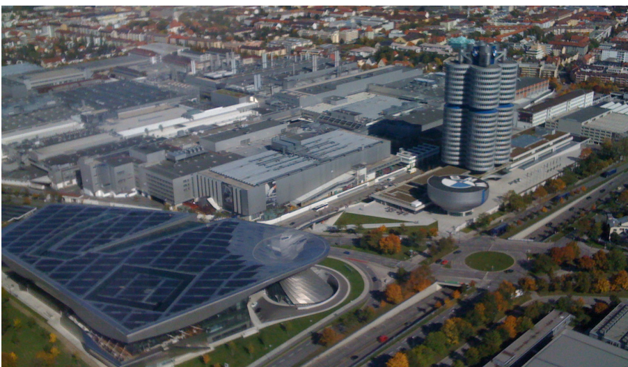
Figure 6: BMW World with solar power installations
