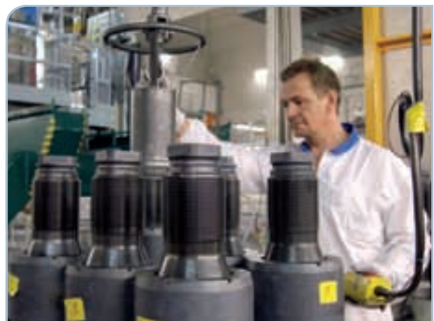
Servicing the bolts of the reactor pressure vessel cover.
