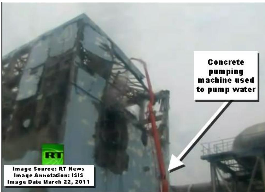
Figure 13. Still from RT News video from March 22, 2011 showing what the Federation of Electric Power Companies of Japan describes as a concrete pumping machine pumping water into the spent fuel pool in the unit 4 building. In the video, see [here](#), a plume of either steam or smoke can be seen rising from the building.
