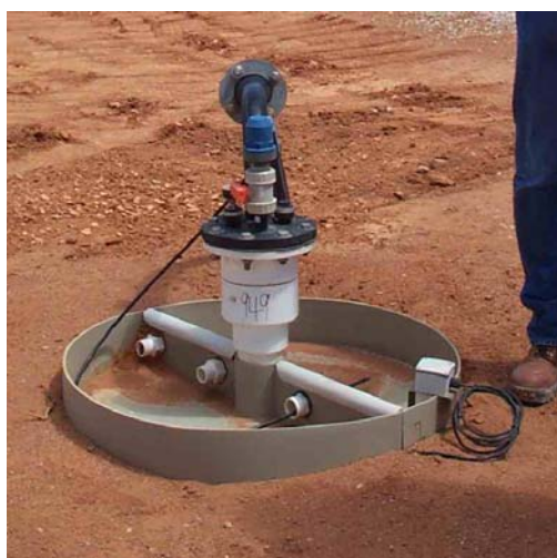
Figure 22 Wellhead with drip tray and online detector, Beverley
