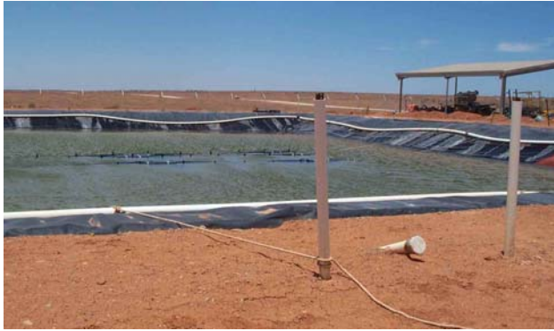
Figure 17 Evaporation/holding pond, Beverley
