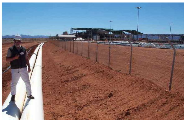
Figure 20 Pipeline from wellfield to processing plant, Beverley
