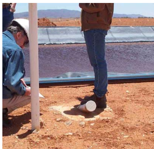
Figure 23 Evaporation pond with leak monitoring, Beverley
