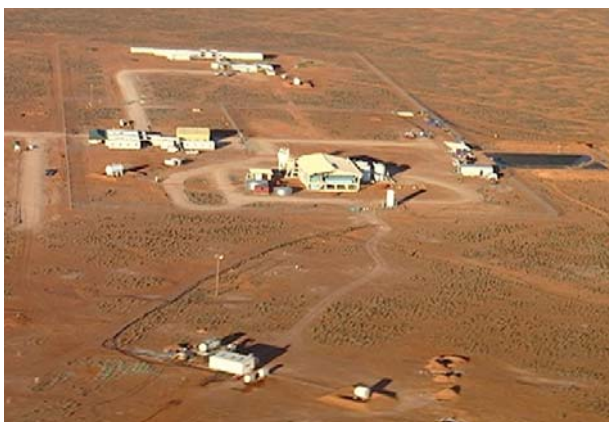
Figure 6 Aerial view of the Honeymoon operation (courtesy Southern Cross Resources)
