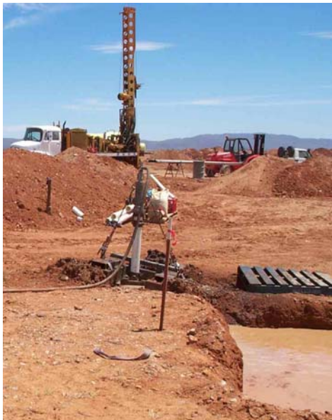
Figure 19 Drill cuttings pit, Beverley
