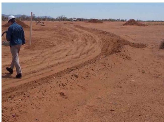
Figure 14 Example of earthen bund, around Beverley wellfield
